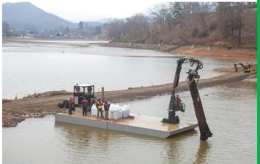
Philip King, of Crestline Global, manipulates the grapple that pulls the log out of one of three gates in the Lake Junaluska dam.
